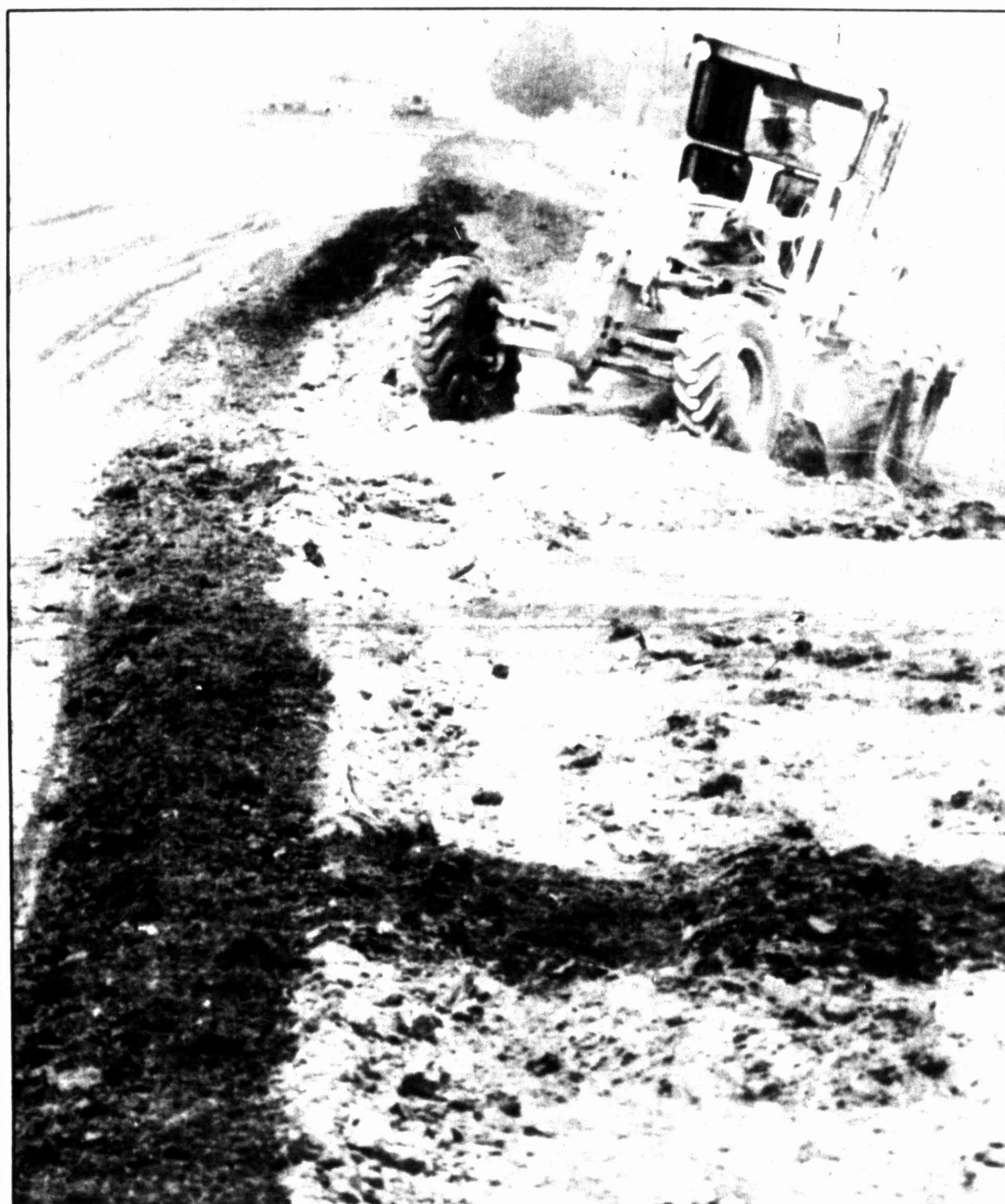
A grader slowly makes its way, spreading dirt along a portion of the miles to be paved as part of the South Highway 87 widening project recently. The road will be converted from two to five lanes from the Garden City Highway cutoff to the Forsan cutoff.
