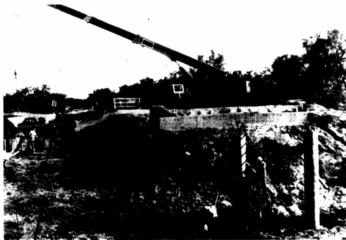
UNDER CONSTRUCTION - Workers are in the process of building one of two new bridges over Morgan Creek in precinct two. The new bridges replaces two iron bridges that were torn down.
