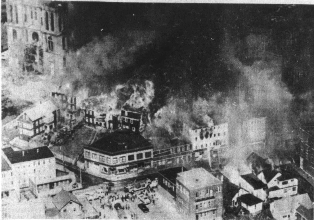
GENERAL ALARM FIRE. A general alarm fire rages out of control in Fall River, Mass., Tuesday afternoon after starting in the Notre Dame Cathedral, upper left, where workmen were remodeling the structure, and
