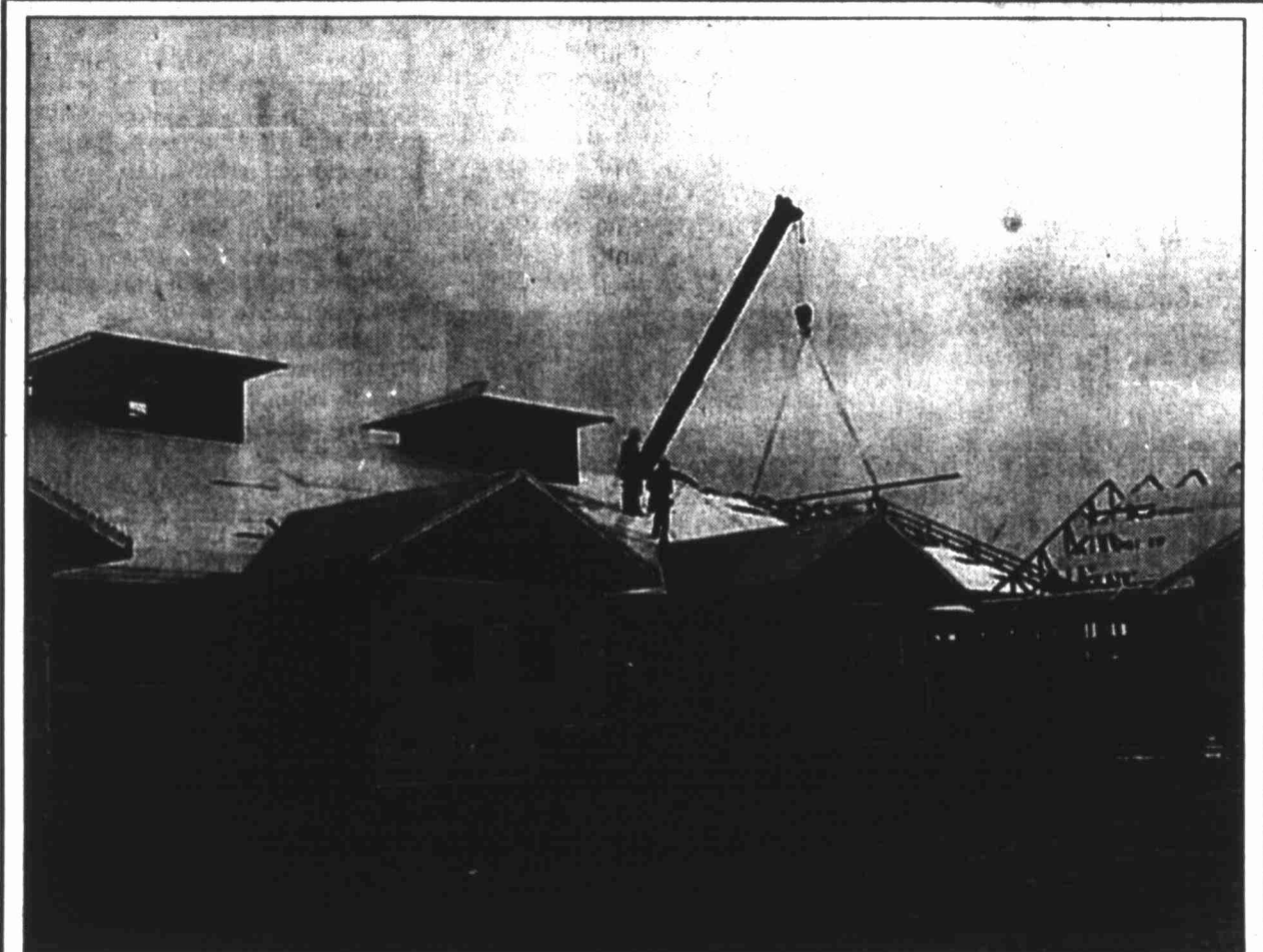
Construction on the State Veterans Home on U.S. Highway 87 is continuing. According to bricklayer Charles Johnson of Mark Young Masonry, the company will lay around 140,000 bricks for the home, which is due completion in October or November.
