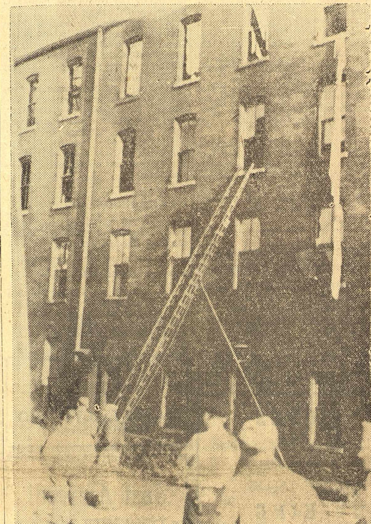
A "blanket ladder", right, swings from the fourth floor of the razed Canfield Hotel in Dubuque, Iowa, following an early morning fire which took the lives of 17 persons. Several guests in the ill-fated hotel used blankets to lower themselves to the second floor level, then dropped, severely injuring themselves.
