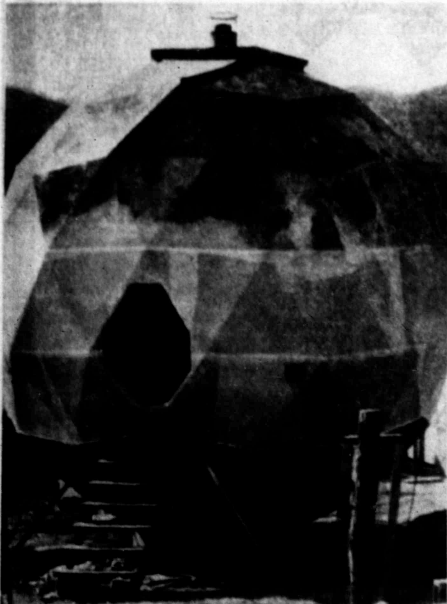
TUCKED AWAY in a mountain valley high in the Blue Ridge Mountains in Roseland, Va., is this modern-day ark—a geodesic dome built by former journalist and Methodist minister Joe Campbell. Campbell says the idea came when his church group discussed catastrophes and noted that legendary survivors all were well prepared. (AP Laserphoto)
