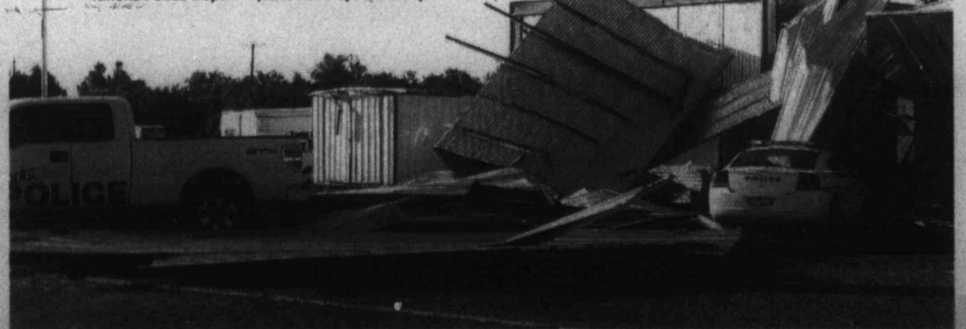
Crunch time ... Metal roof comes crashing down on Tahoka Police Dept. (LCN PHOTO by Pam Elrod)
