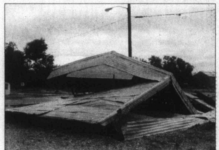
All came tumbling down ... This metal barn on Lockwood, near the eastern edge of Tahoka, was destroyed during Saturday night's thunderstorm, from apparently high winds.
