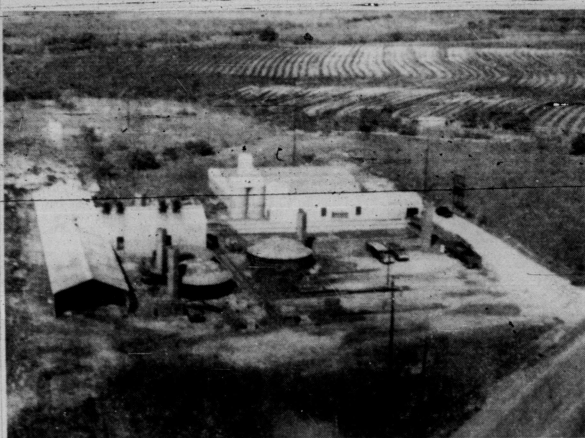
THIS IS THE PLANT of Southwestern Brick and Tile Co. just southeast of Snyder where the raw clay from a pit on the Hugh Mason Ranch is turned into brick and tile products. The products of the firm are used not only in Snyder, but over a wide area including East Texas, New Mexico and Oklahoma.
