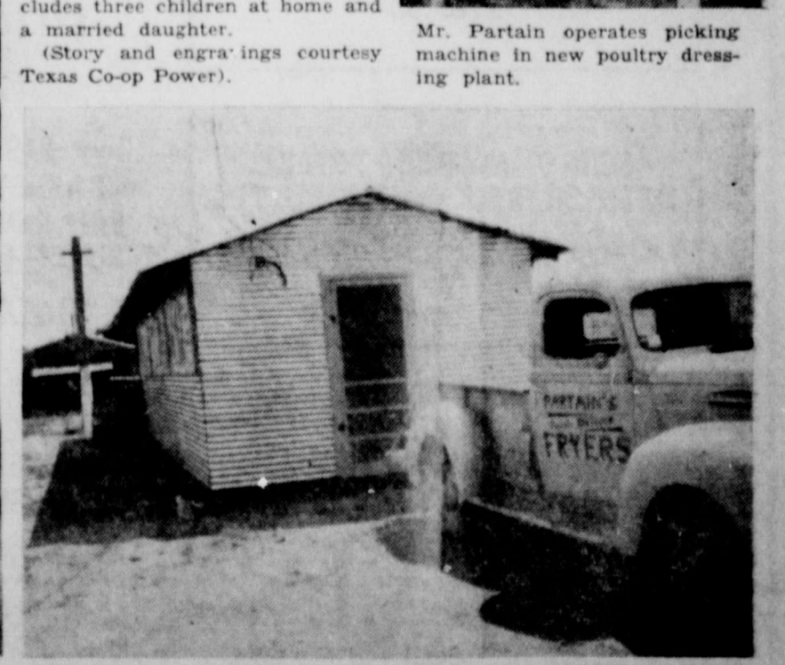
Partain's poultry dressing plant with poultry houses in background.
