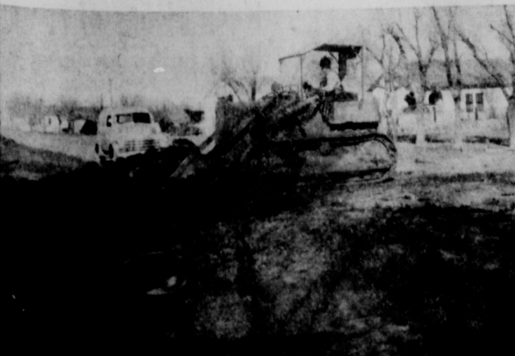
PAVING WORK—The city maintenance workers have been busy the past week replacing culverts and digging ditches on S. Ash street for better water drainage, if and when it rains enough to make water a problem. Above is Milton Freeman with the city tractor loader at work on the intersection of 4th and 8th avenue.
