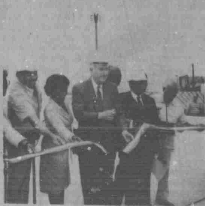
GLORIOUS DAY -- Pictured are a few of the hundreds of citizens who participated in the historic ribbon cutting of the East 34th & Quirt overpass. More than 300 person were in attendance. At left, Mayor B. C. "Peck" McMinn is shown cutting the ribbon, along with other citizens, including Rev. Kado Lang, chairman of the
