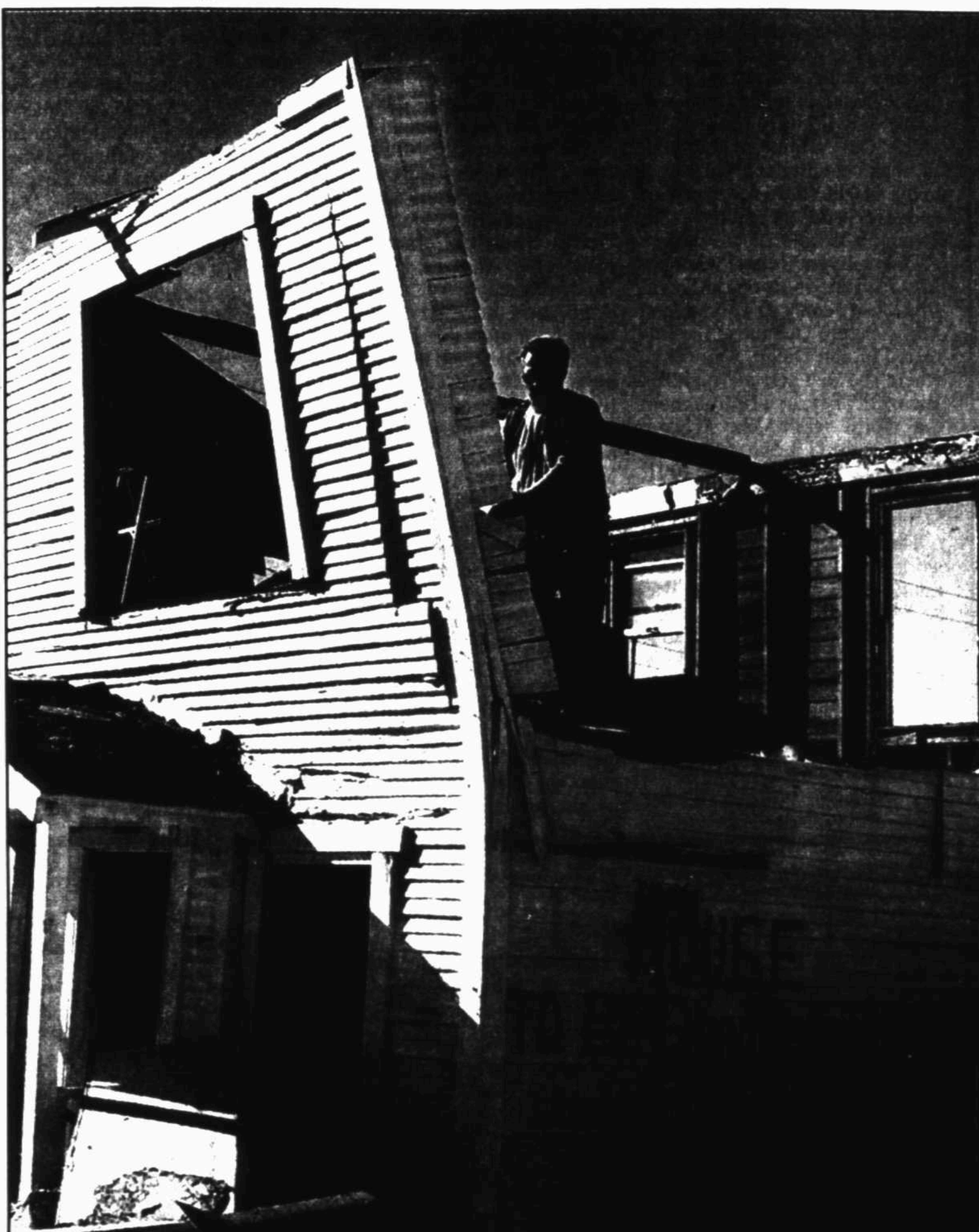
Dennis Clements works on tearing down part of his house at 507 N. A St. Monday morning. The city condemned the building and required that it be torn down. This is the second property Clements owns the city has condemned.
