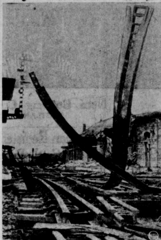
Tortured into twisted scrap iron, these rails show how railroads, vital links in army communications chain, were smashed. The photo above shows the Jemelle, France, railroad station, after Nazi bombers scored direct hits.
