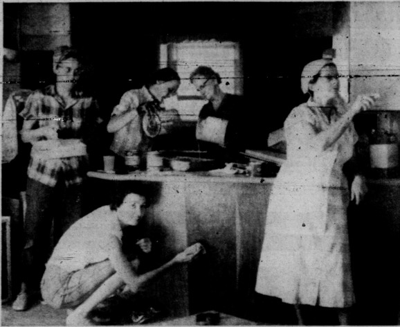
PAINT UP, FIX UP —Members of the Fluvanna Church of Christ are going full steam this week painting, finishing and air-conditioning a home for their minister, Roy Pheaster who will move to Fluvanna from Big Spring when the building is ready. Working on the painting and getting paint refills here are Mrs. Sandy Holder, Mrs. C. T. Hunnicutt, Mrs. H. C. Carmichael, Mrs. C. A. Dougherty, and Mrs. C. N. Ainsworth.
