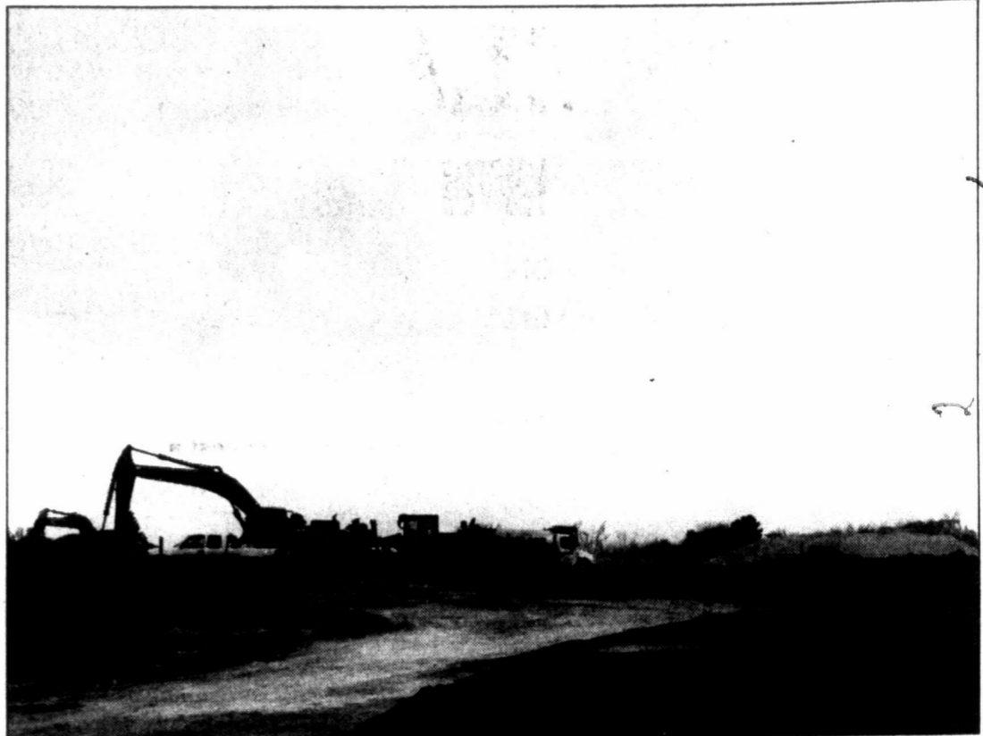
ON THE MOVE - Preliminary construction work is continuing on the new Colorado ISD K-8 campus near the high school. Workers completed the installation of drainage pipe under 10 th Street last week and reopened the street to traffic.
