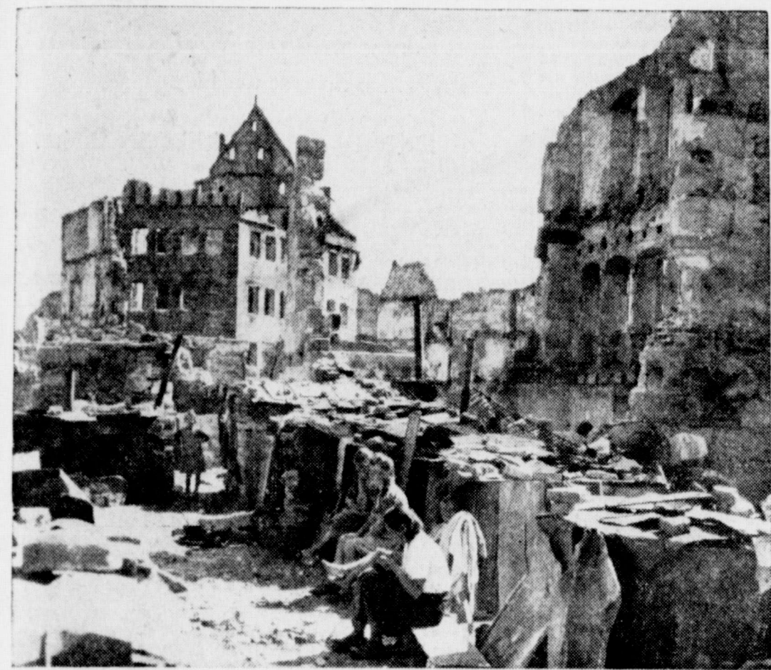
POSTWAR GERMANY—As shattered as Hitler's promises are the hopes of residents of Nuremberg for early reconstruction of their homes. Buildings bombed by Allied planes are empty skeletons. Townfolk sit dejectedly beside sheds. Air raids shelters are the only roofs.
