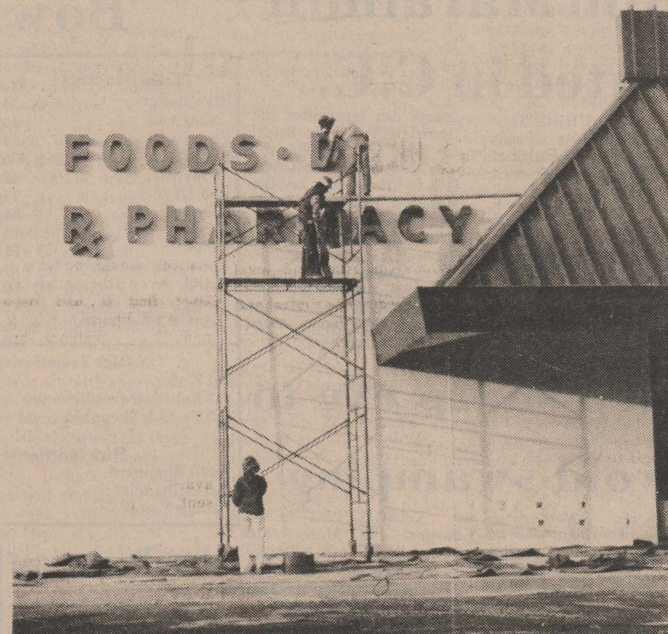
WORKERS INSTALL signs on the new H.E.B. store being built in Rockport. The store is scheduled to open in mid summer and is on schedule. [Pilot photo by Ted Norman]
