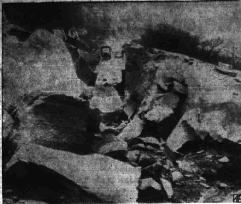
ROAD CLOSED —Tons of rock covered 200 feet of state highway 7, Skyline Drive, near Marietta, Ohio. The rock slipped over the road, which was cut through almost solid rock a few years ago. No one was injured. Highway engineers said the road would be closed for two or three days. (AP Wirephoto).
