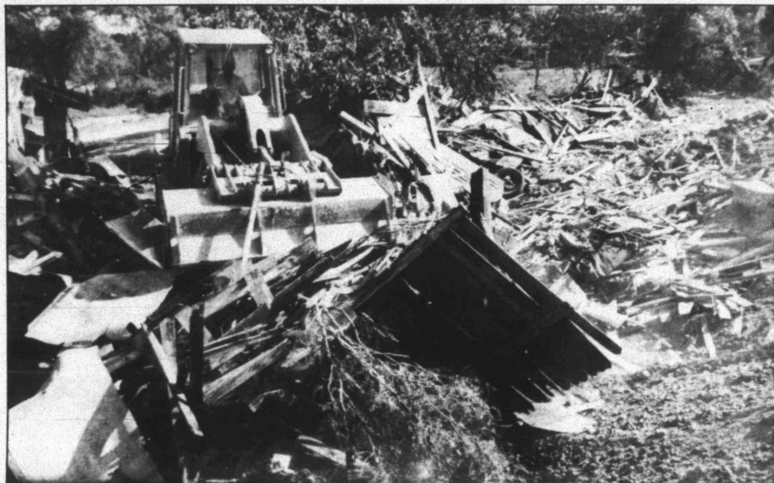
Shoving debris away
