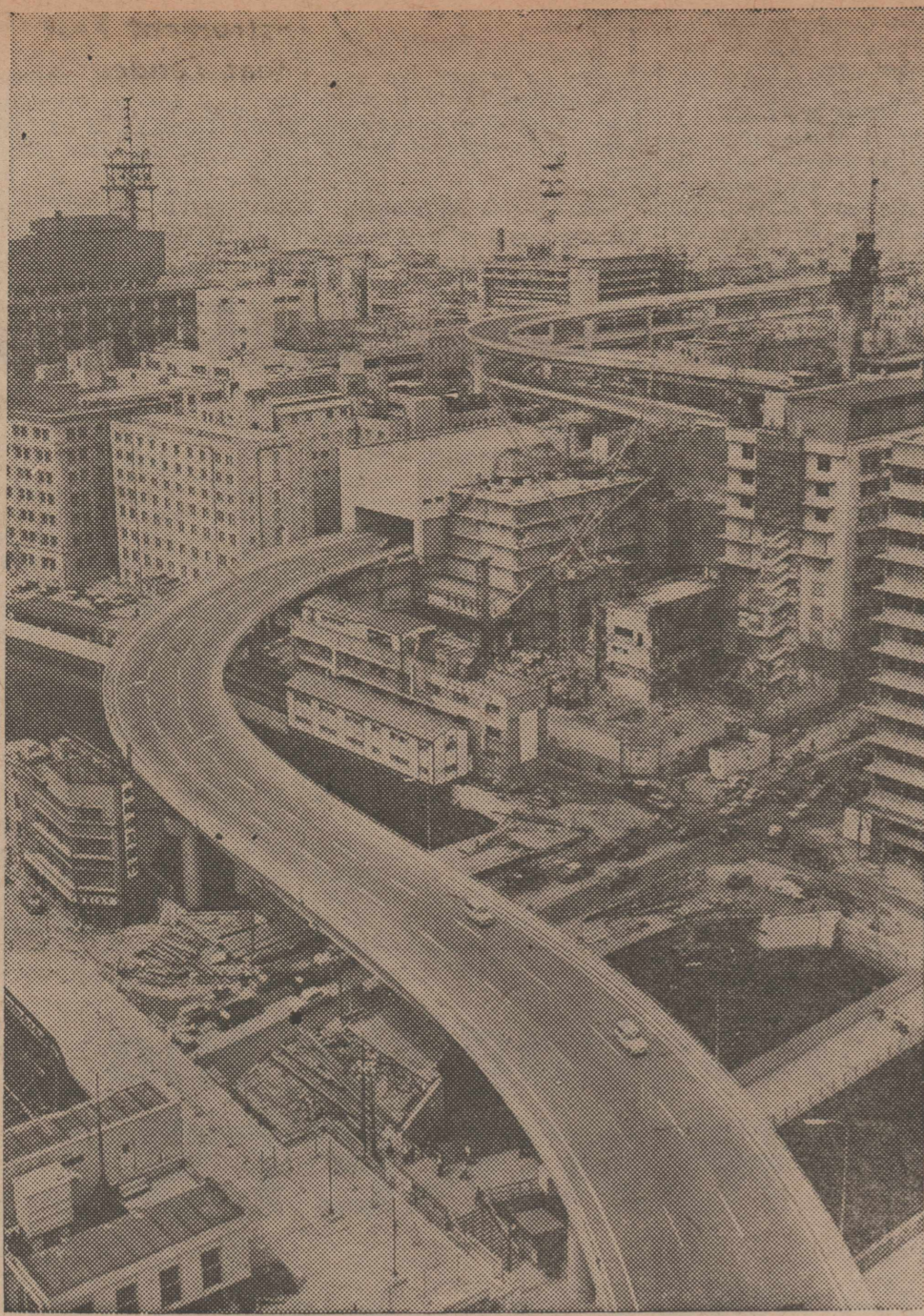
EXPRESS HIGHWAYS curve and cross over the river in downtown Osaka, where an increasing number of modern office buildings attest to the growth of Japan's second largest city. The coming of Expo '70 has sparked even more construction.
