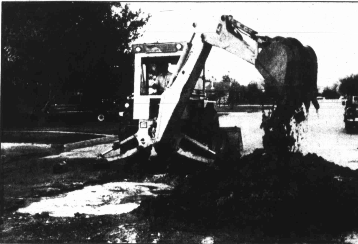
Working on broken water line
