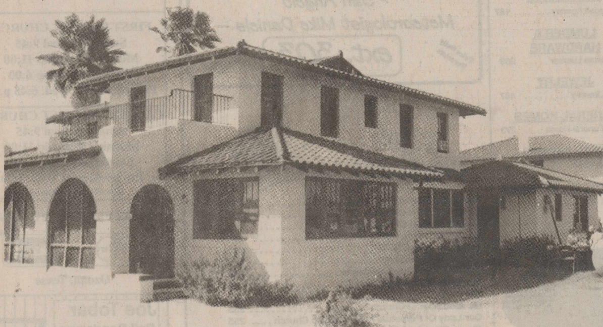
THIS NORTHEAST VIEW of the O. W. Parker Ranch Headquarters house is a good example of the Spanish Colonial Revival architecture. The Parker Ranch Headquarters was dedicated Oct. 28 as a Texas Historical Site.
