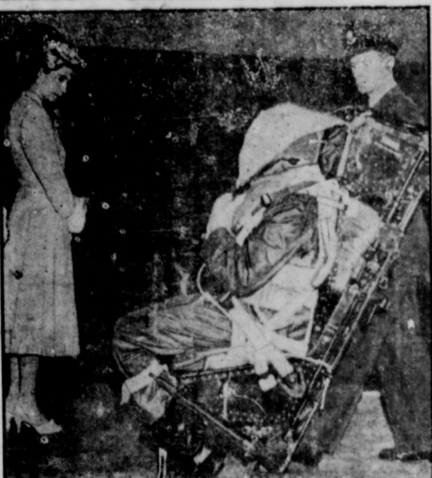
HOW SHY CAN ONE GET?—To stare at a queen is one thing—to be stared at by Britain's Queen Elizabeth is something else again. However, the "shy" airman hiding his face isn't overcome by the experience. He's demonstrating the action of an ejection seat canopy which shields a pilot's face when the must bail out from jet aircraft at speeds in the near-supersonic range. Her Majesty was treated to the demonstration while touring an air base at Marham, Norfolk, England.
