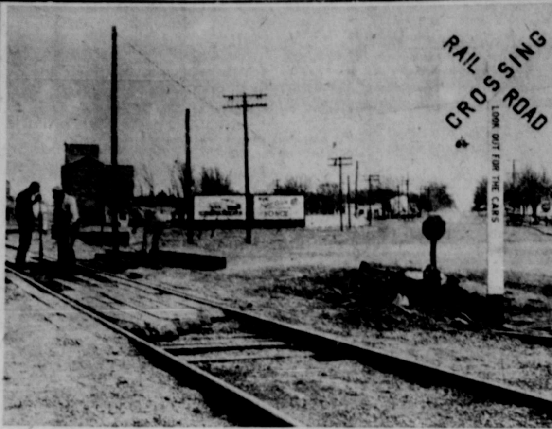
NEW CROSSING—These three Santa Fe employees are shown putting in new ties for an improved railroad crossing on 3rd avenue. The new crossing is being done by the Santa Fe while the city is improving the pavement on the road leading to the fair grounds. Above are Ernest S. Parker, Rufus Hickey and Harry Karnes of the Santa Fe.
