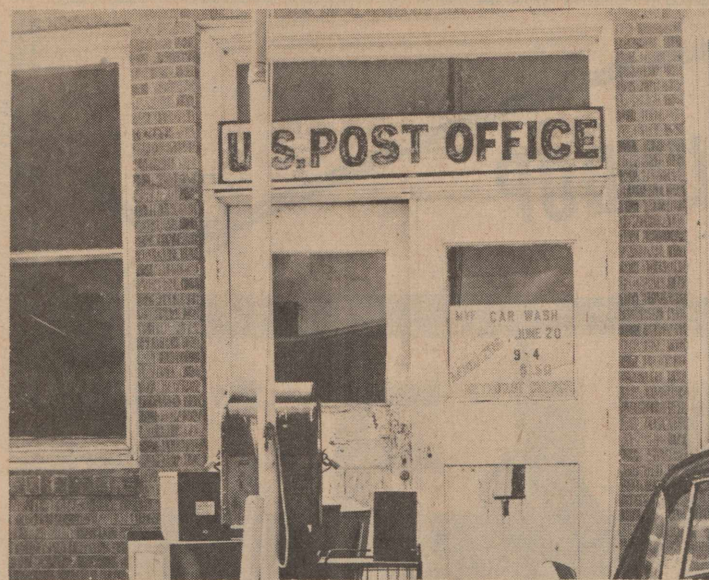
OLD POST OFFICE BUILDING
