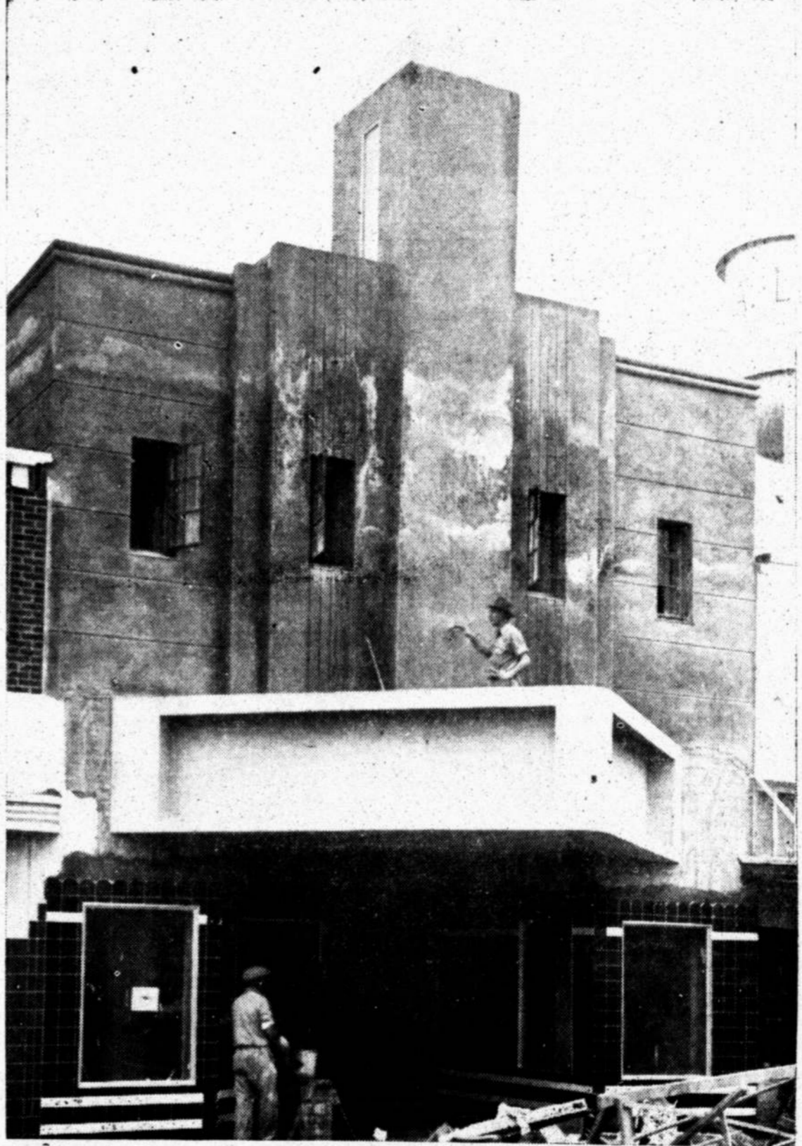
Scene showing Tower Theatre under construction
