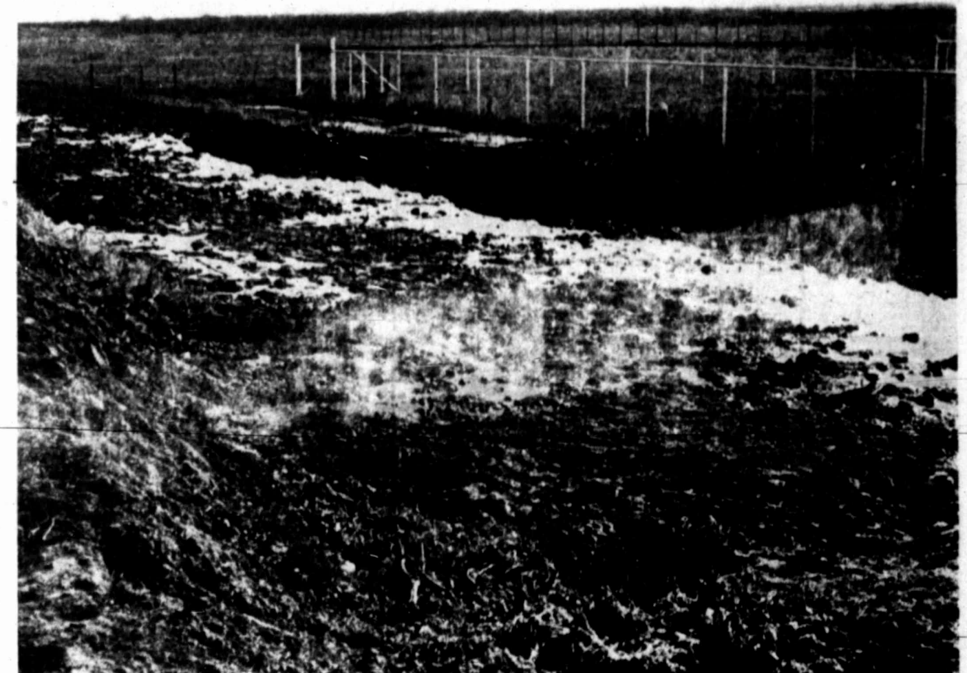
Sewage and water stand atop the new drain field at Midland Mobile Home Ranch.
