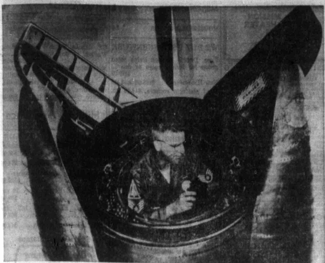
The Pipe Gets A Check
