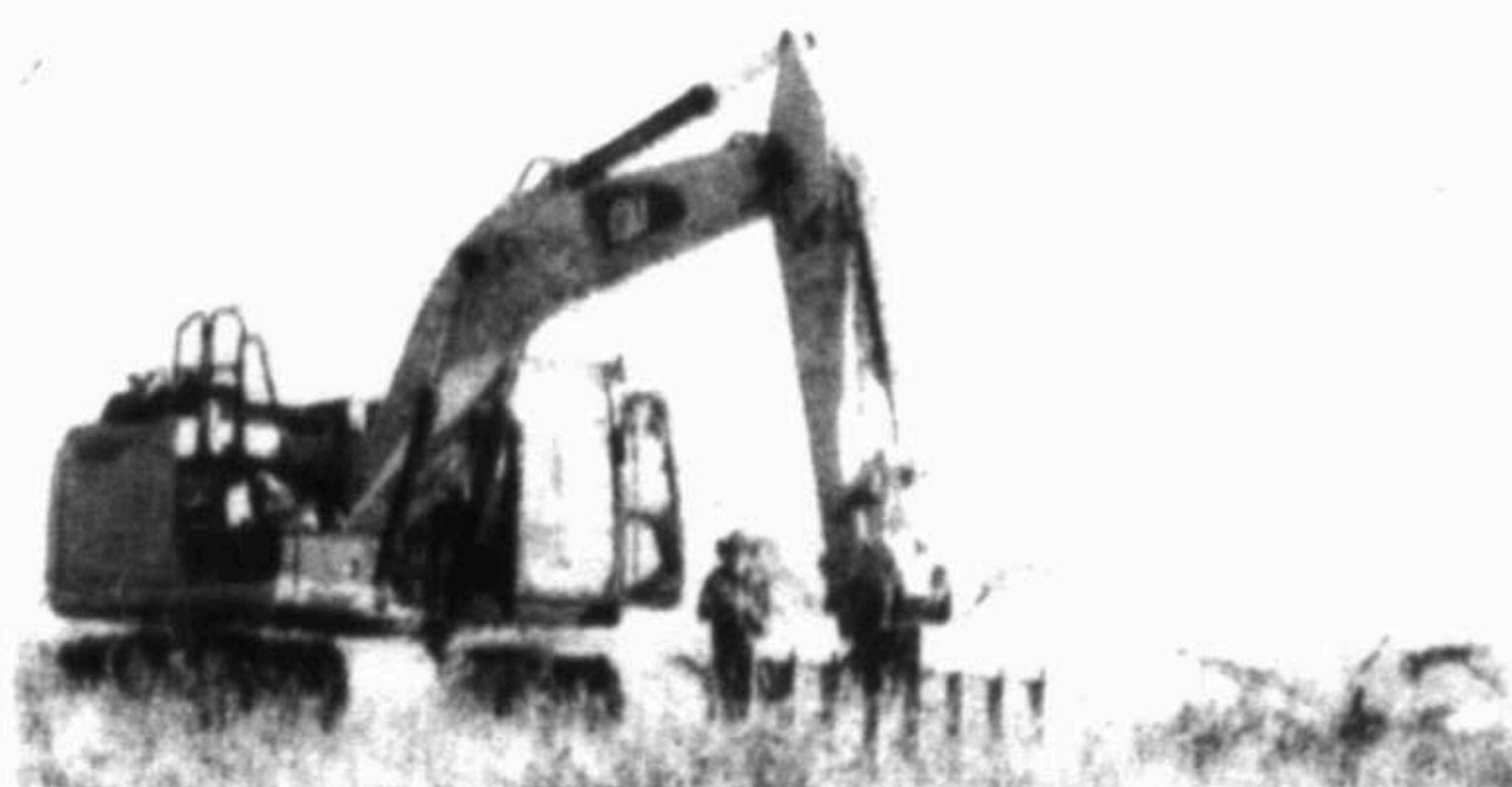
The right machines operated by trained, dedicated, local personnel means grubbing and leveling are done right, preparing land for the pads, roads and fences that are part of the drilling and production process. Call John Evridge at Anderson Grubbing Services, 432-556-5241.
