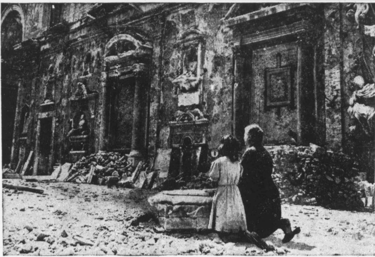
FAITH IS INDESTRUCTIBLE . . . The beautiful cathedral at Leghorn, Italy, ravaged by the war, is now little more than the spirit of a place of worship. Some of the debris has been cleared up, and all that was salvagable was saved for use in reconstruction. Meanwhile, the people continue to go to the ruins to pray as they always did, for neither bombs nor shells nor the destruction of their cathedral could dent their faith.
