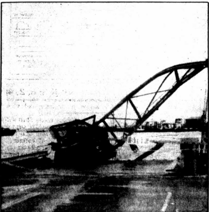
A barge moves through the Houston Ship Channel past the twisted wreckage of the Lynchburg Ferry's south landing in Houston. A barge accident caused the closure of the ferry landing for several months, forcing commuters from east-side suburbs to use alternate routes into Houston.
