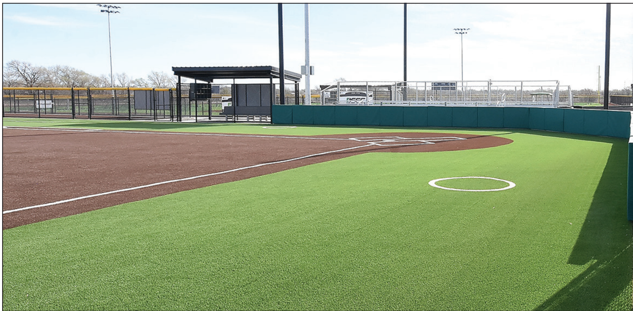
Ribbon Cutting — Hereford City Commissioner Deven Black invited the Friona Star to attend the Ribbon Cutting for the new multi-million dollar John Bunch Sports Complex in Hereford on Saturday, March 29th. Mayor Cathy Bunch cut the ribbon for the new facility which features 4 baseball fields covered entirely in field turf. Over 1,000 Hereford residents attended the event. Caviness Beef Packers Company served free hamburgers to all attendees. Deven is a 1994 FHS graduate and former Friona resident. He and his wife, Melissa, live and work in Hereford. Melissa also works in the lab at Parmer Medical Center.
