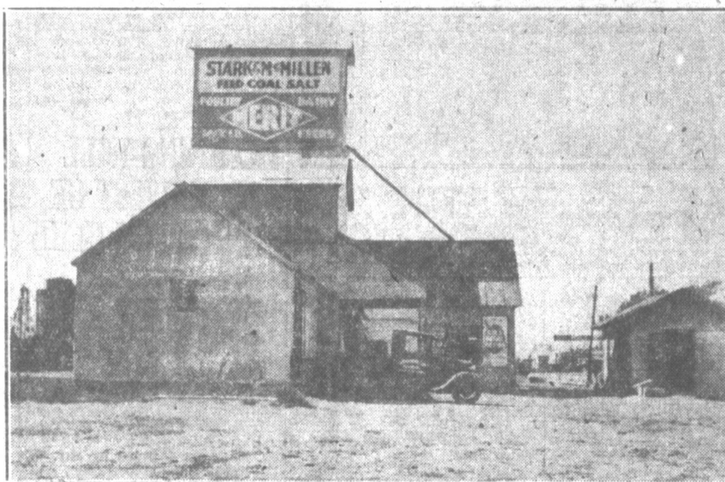
Stark and McMillen Elevator and Warehouse
