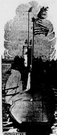
Uncle Sam's greatest submarine, 34 1/2 feet over all, just launched at Portsmouth. She is nearly twice the size of any other under-sea craft and can travel 21 knots an hour on the surface or 9 knots an hour under water. She is fast enough to stay with major ships during maneuvers.
