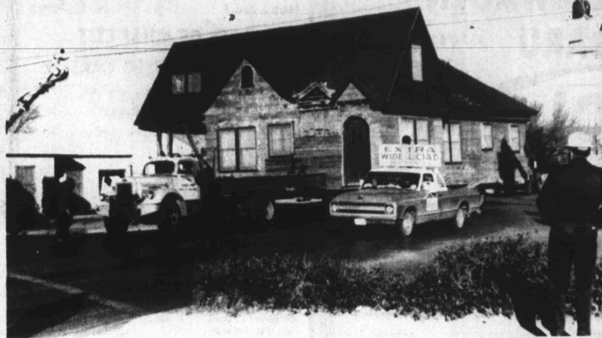
BEWARE: HOUSE CROSSING — No, this is not Howard Hughes' Winnebago. This is a somewhat slower process than Dorothy's trip over the rainbow, but nonetheless, this house will get moved from 702 Goliad to Forsan with the help of utility and city employees. Be it ever so humble...
