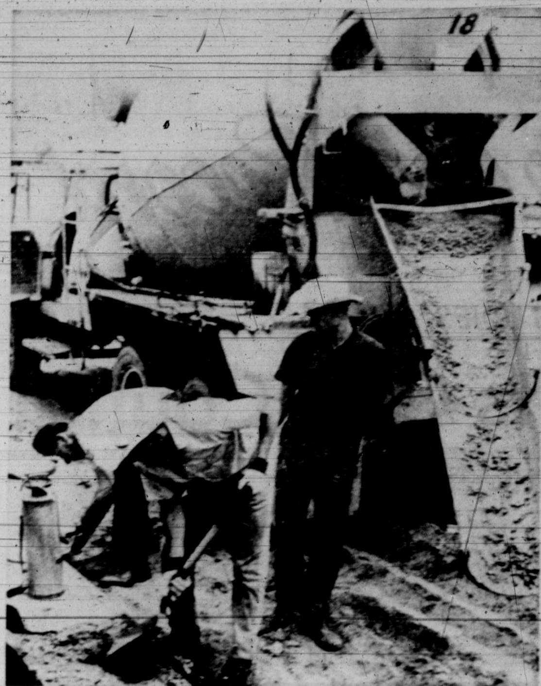
Paving Job To 17th Street
