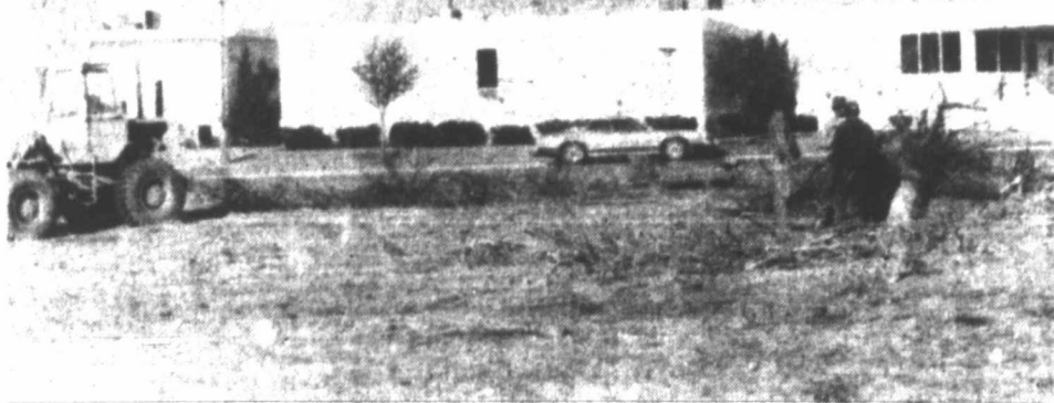
VISITORS AT ROOT MEMORIAL HOSPITAL and Valley Fair Lodge will no longer have to worry about a place to park as construction on additional parking space got underway Tuesday. The new parking lot is located east of the hospital on Chestnut.
