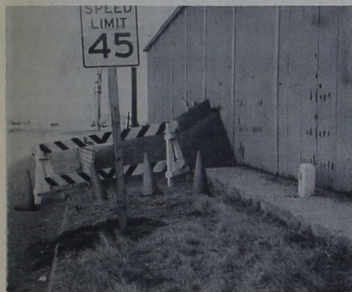
A RUNAWAY HORSE TRAILER hit the side of Bovina Wheat Growers grain storage building on Highway 60 Saturday afternoon, knocking a hole in the side. About 20,000 pounds of grain spilled through the hole and approximately $1,000 damage was done to the building, according to a spokesman at the elevator. Aaron Drager of Texico was pulling the horse trailer when he hit the dip in the highway in front of Bovina Restaurant, causing the trailer to come loose from the pickup.
