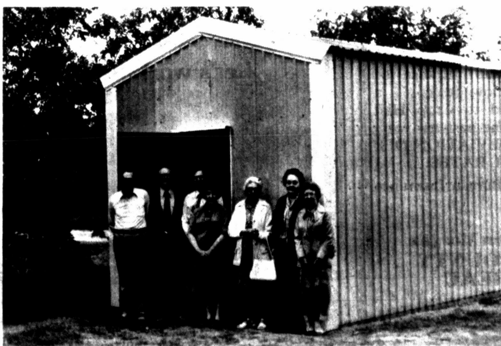
A FEW OF WOODLAND SCHOOL board of directors gather in front of the new newspaper building built by RASP Construction Company. Shown are (front) Elmer Martin, Roger Wells, Kenneth Rogers, Marion Bassham, Dona Reed, Cecile Smith and Mrs. Bruce Johnson of Loraine.
