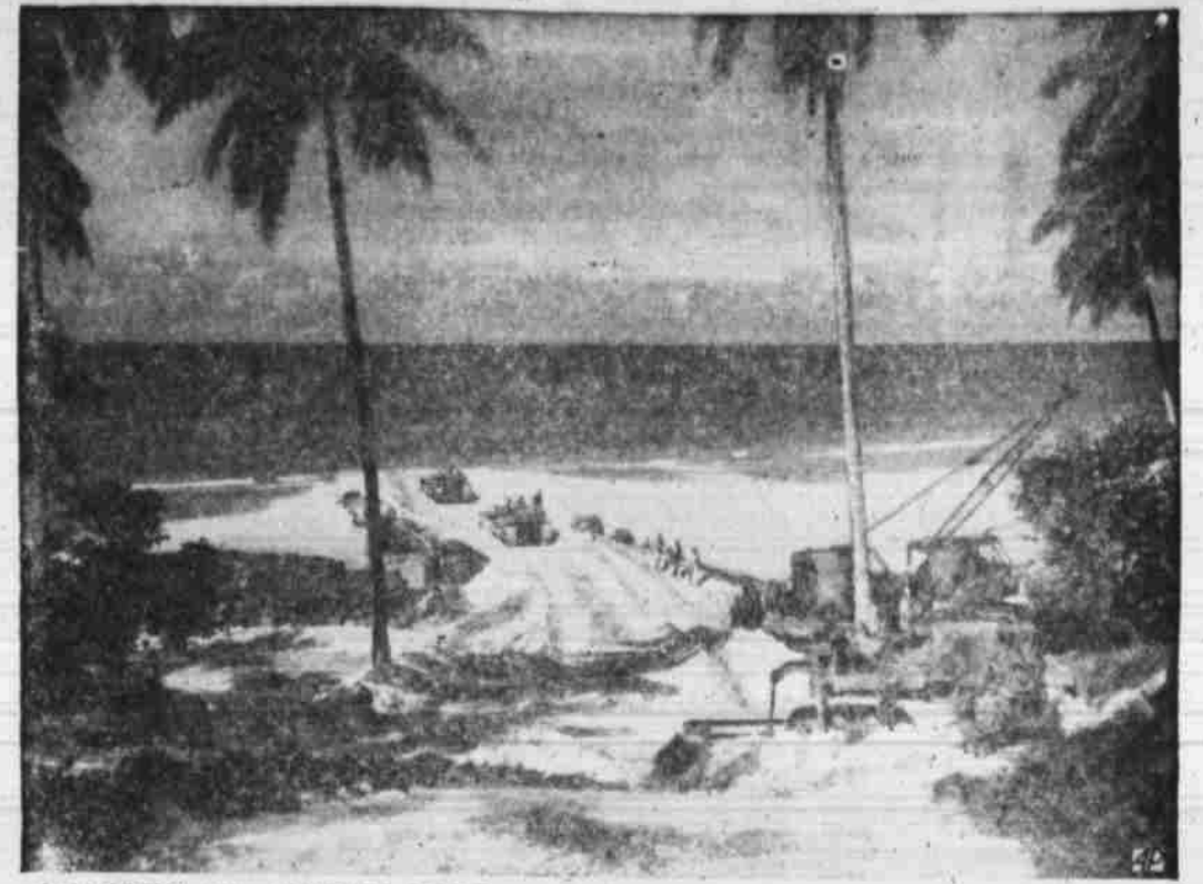
SEABEES IN SOUTH SEAS —Using bulldozers, U. S. Navy Seabees clear a road to a dock site on Emirau Island to facilitate unloading of LSTs.
