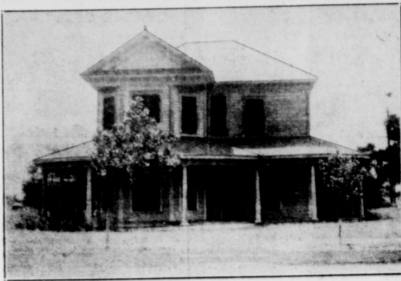
A home that for many years served Burkburnett people is being torn down to make room for a modern brick building to house the Owens-Brumley Funeral home.
