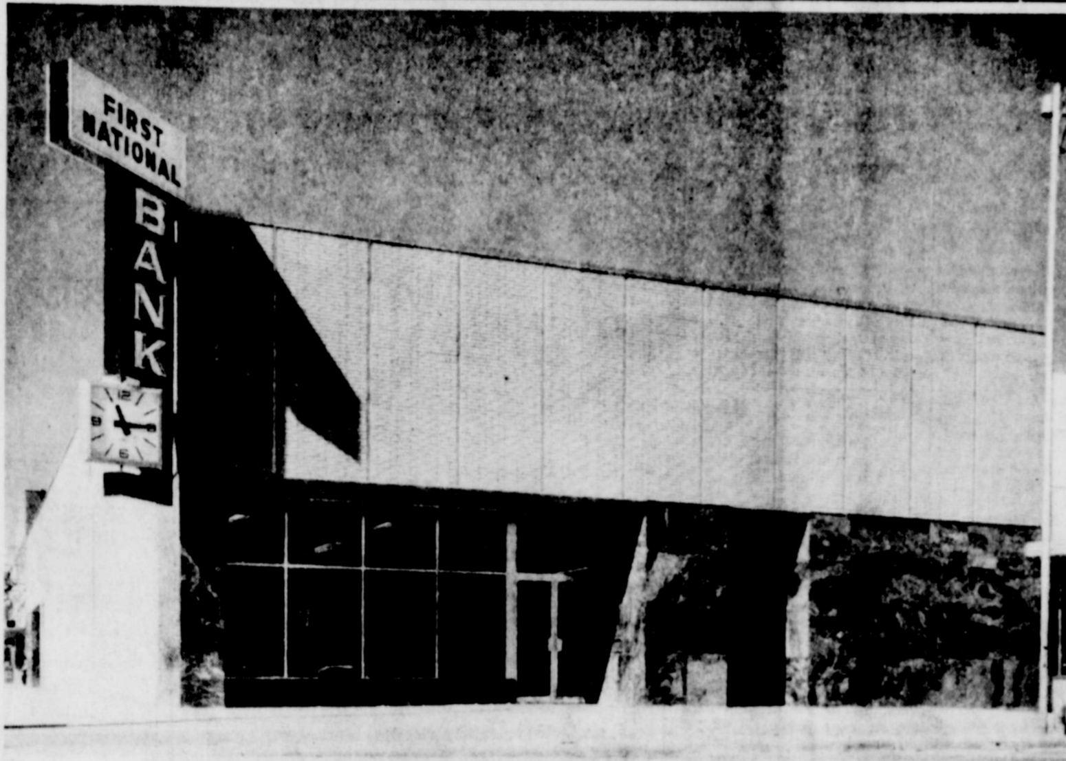
The new First National Bank which will be opened to the public at an open house Sunday afternoon and open for business Monday morning, is pictured above. It has taken almost a year of planning and building. In dollars and cents it represents an outlay of slightly more than $175,000, but the finished product is the most modern banking facility on the South Plains.
