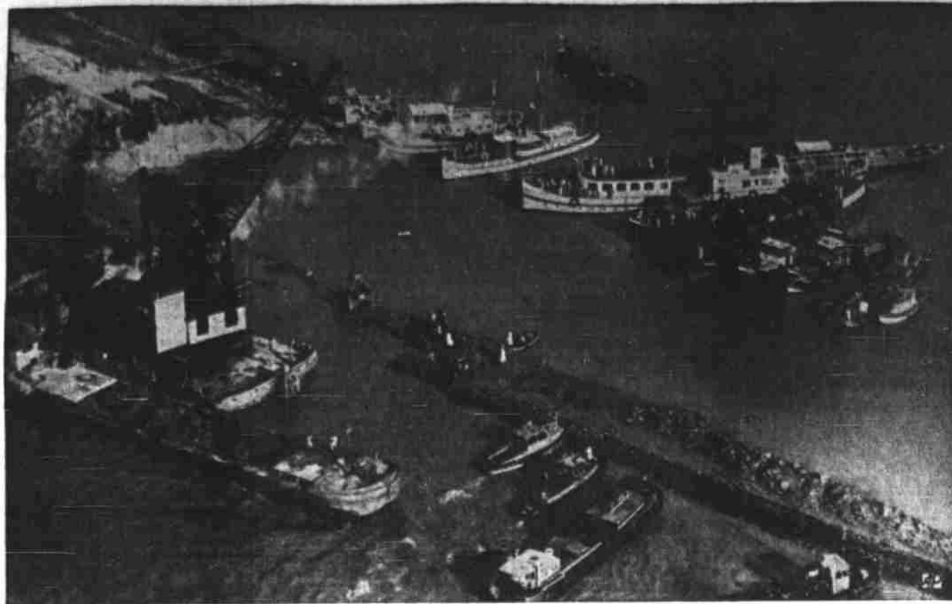
OPENING A NEW PROVINCE IN HOLLAND — A marine "gallery" is on hand as crane closes the last opening in Holland's new 15-mile dike leading to reclamation of the future 500,000-acre Zuider Zee Province.
