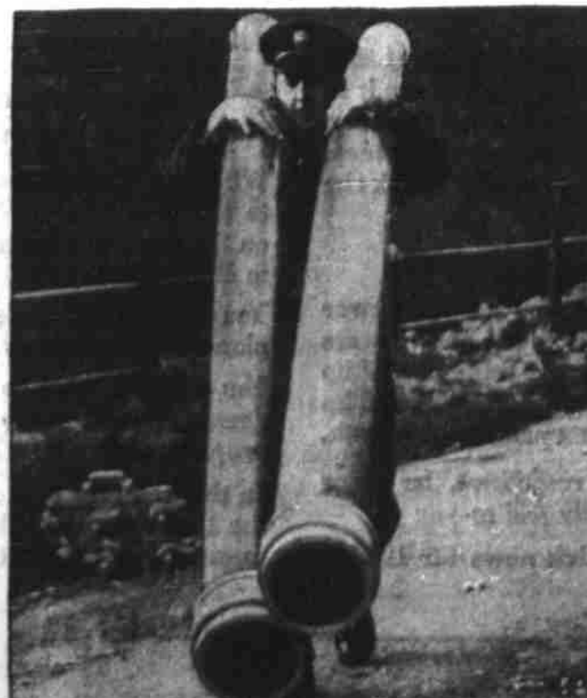
FOR FASTER FIREFIGHTING — A Kent, England, fireman carries two 16-foot lengths of lightweight plastic pipe during a demonstration of high speed firefighting.
