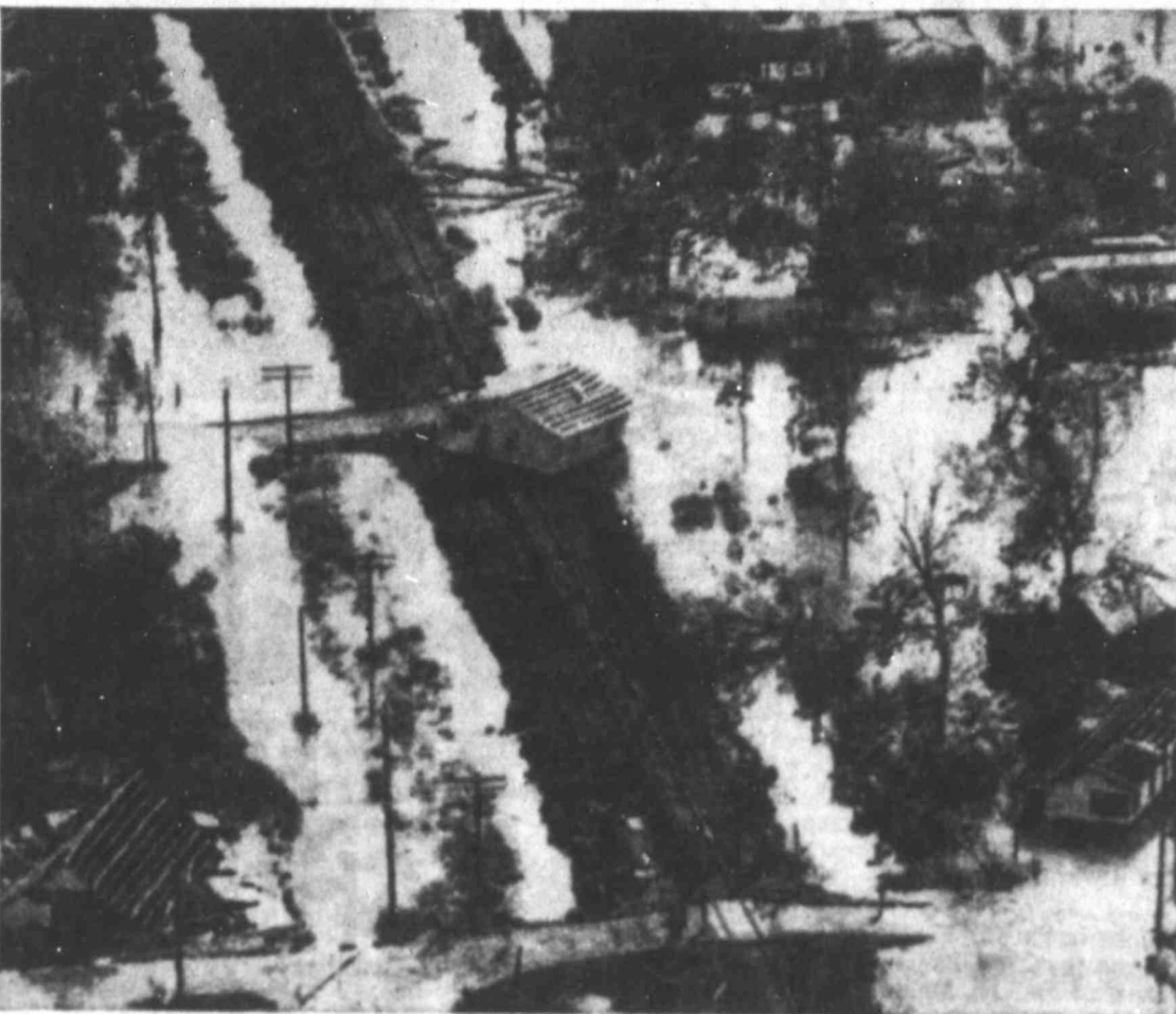
CAMILLE DAMAGE—Hurricane Camille which struck the coast of Mississippi early this morning picked up a huge house from its foundation and dropped it on train tracks between Gulfport and New Orleans. Winds of 150 miles per hour hit the coast.
