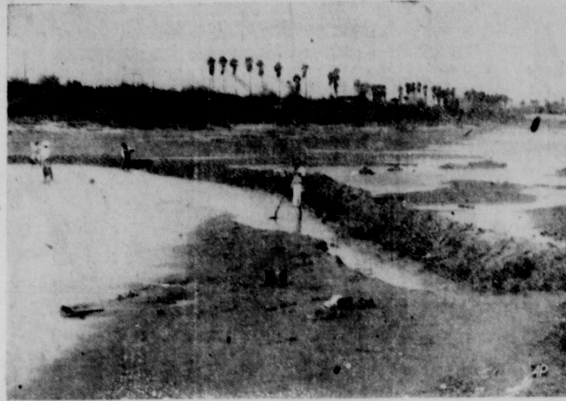
EARTHEN DAM STIRS PROTESTS —Farmers of the arid vegetable growing area south of Brownsville, Tex., have protested against this earthen dam constructed across the Rio Grande by Mexican workers. The Laborers built the dam to divert water from the river to Matamoros, suffering badly from lack of water. Farm officials say 100,000 acres of crops are endangered by the long severe drought which hit the Valley and northern Mexico especially hard. (AP Photo)
