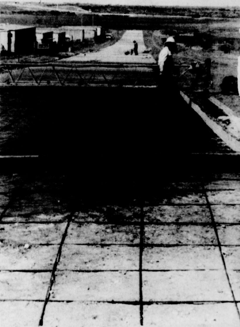
WORKING ON ENTRANCE WAY TO THE WALLACE UNIT: One of the last projects started at the 80-John Wallace Unit was the entrance road to the unit. It is located on the northside of the unit off Rogers Road.
