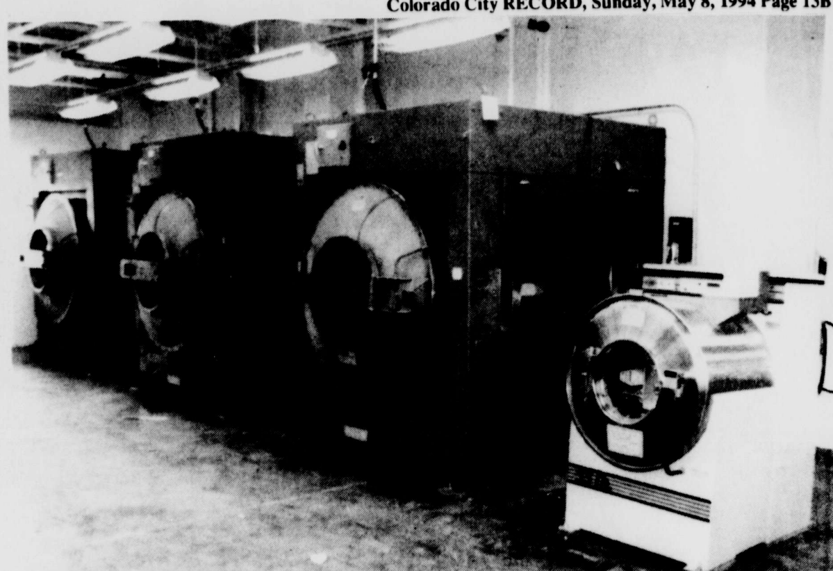
Washers in laundry room
