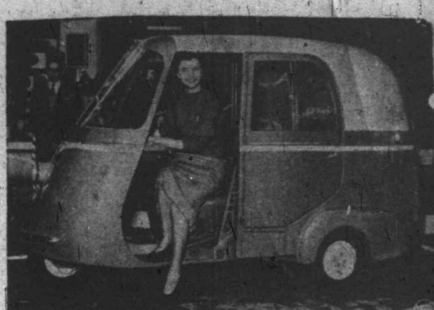
TINY TAXI —A model lends a decorative touch to the otherwise utilitarian "Micro-Taxi" just unveiled at the Milan, Italy, Industry Fair. The three-wheeled midget taxi, designed for two passengers, is really a motor scooter with a special housing. Designer claims it offers lower fares, good speed and gas-saving mileage.
