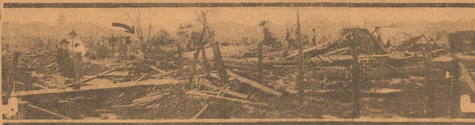
The above photo shows what was left of seventeen homes on the Enterprise Road, about one mile south of Meridian, Miss., struck by the tornado that swept sections of northeast Mississippi, north-west Alabama and southern Tennessee last week, taking a toll of more than 100 lives. Arrow points to the site of the home of H. F. Eastburn, whose wife and three children were killed.
