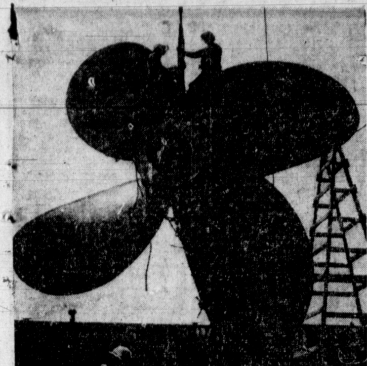
TOP PROP —The largest propeller ever installed in a ship dwarfs the workmen riding it at Newport News, Va. The 73,000-pound propeller is 24 feet in diameter. It was installed in the 810-foot, 60,000-ton tanker Salsimena.
