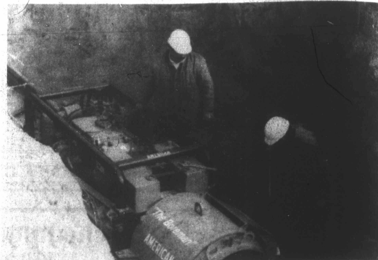
Construction is well under-way on the new water line being constructed for the new prison. Construction workers bore the first of two lines under Rogers Road last Wednesday. It takes less than a day to bore the 16" line.
